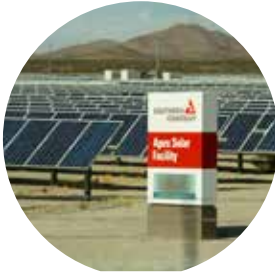
Apex Nevada Solar LLC
