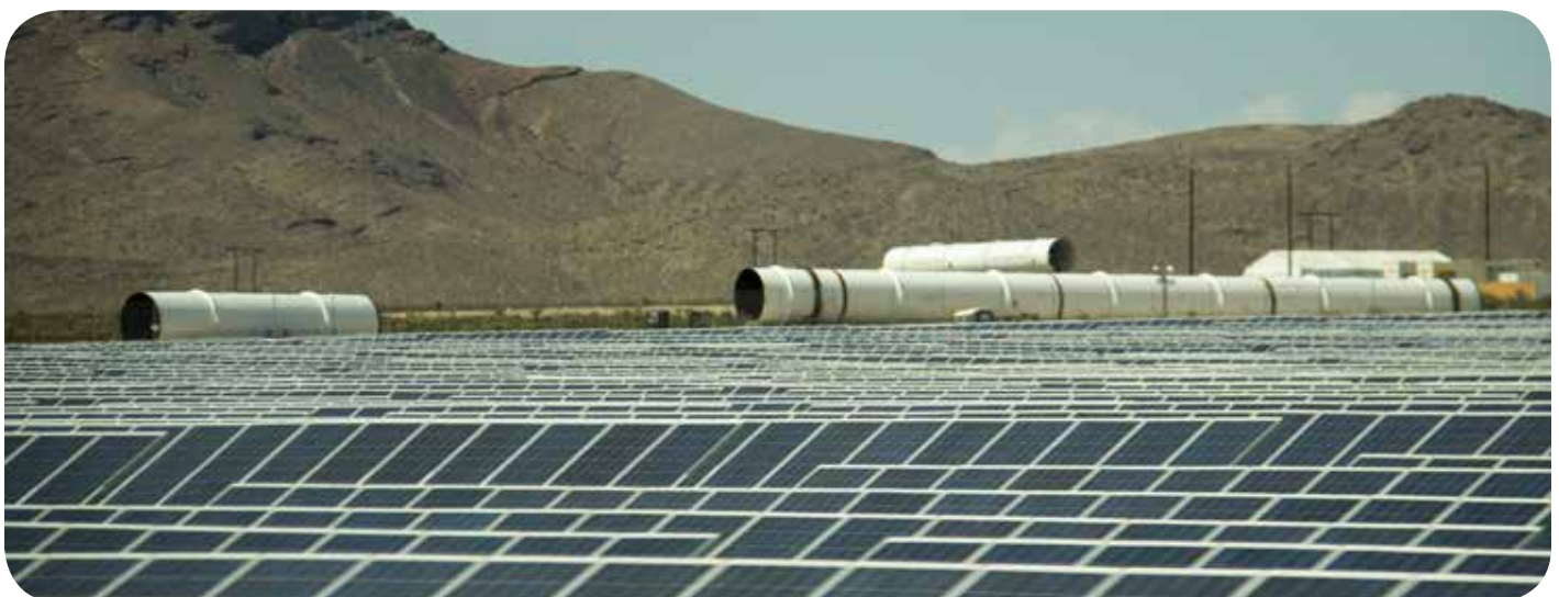
Hyperloop Test Tubes and solar energy, the sustainability technology of today and tomorrow are in operation at APEX
