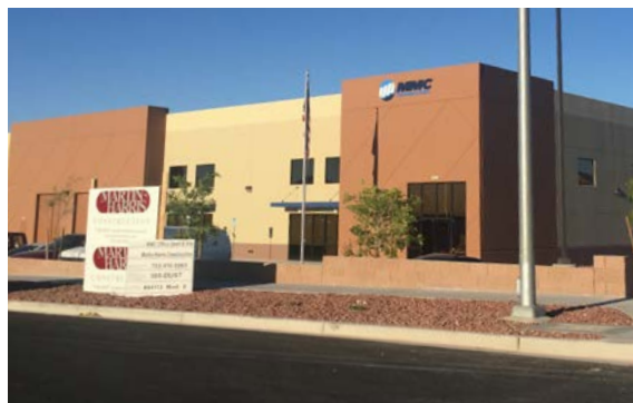
PHOTO – MMC Contractors is an employee-owned company located at 7040 Redwood St. and specializes in large, complex mechanical projects, with a comprehensive offering of pre-construction and construction services.
